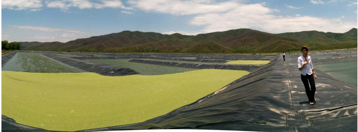
Partial view of one of the ideal 30 has, plug-flow, tropical wastewater treatment lagoons in Salta.
